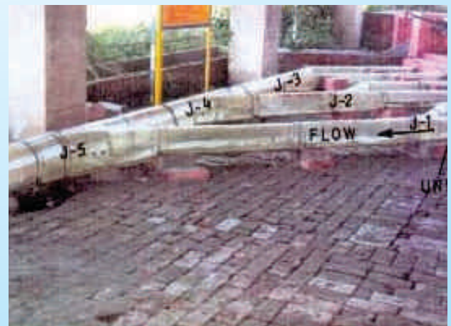
Water Conductor System of Tala HEP, Bhutan
